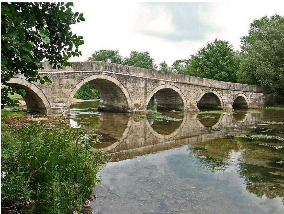
Fig. 9. Stone bridge construction at Plandište near Blažuj (Sarajevo surroundings)
