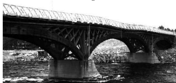
Fig.11.1 Historic wooden bridge of the Oulu River
