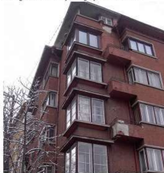
Sofia. Building cooperative with a constructivist vision, 1934.
