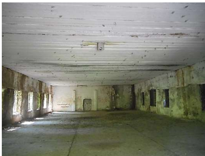
Fig. 10 View of the ceiling with pre-tensioned beams and concrete topping (own photo)
