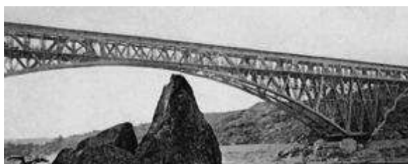
Fig. 20.4 Kichkas bridge across the Dnipro, 1902
