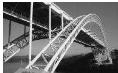
Fig. 24.7 New Saikai Bridge
