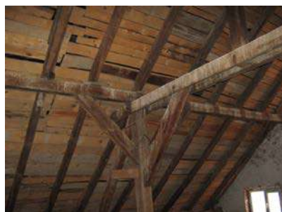
Fig. 3.9. Connection between column, purlins, pliers and struts on the second level of the roof
