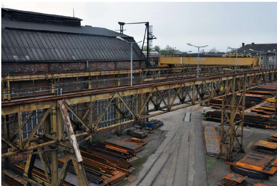
Fig. 2. Overall view of analyzed steel truss structure
