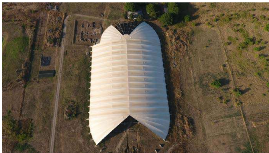
Fig. 2 The first phase of construction of the protective structure (2015)
