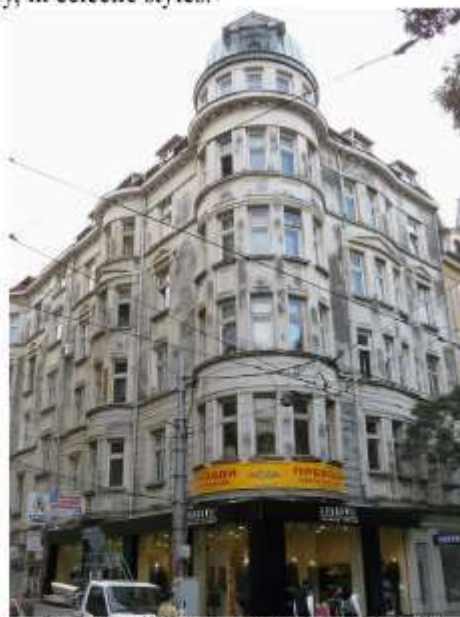
Sofia. Building cooperative "Globe". Beginning of the 1920s (architectural bureau Nachev-Fingov-Apostolov) with a built-in two-story building from 1912 (arch. Nikola Lazarov).
