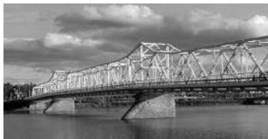
Fig. 11.2 Tornio River Bridge, built in 1939.
