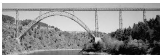
Fig. 12.1 The Garabit viaduct, designed by G.Eiffel
