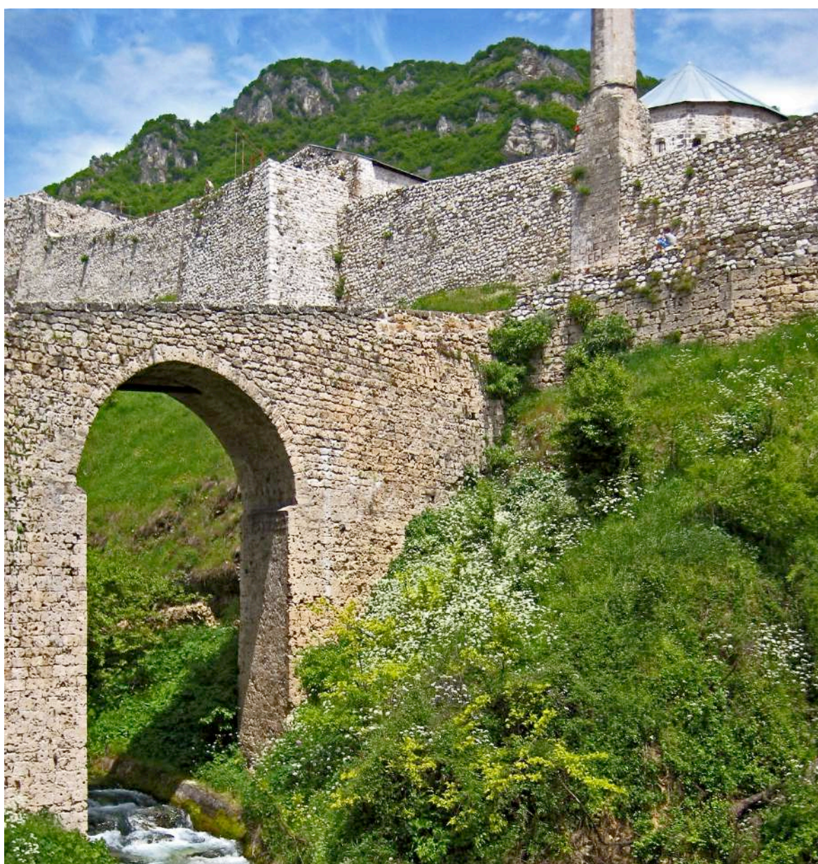
Fig. 8. Stone bridge construction where the wooden construction of parapet was subsequently replaced with a walled korkaluk (parapet). Entrance into the Old Town in Travnik from the west side.
