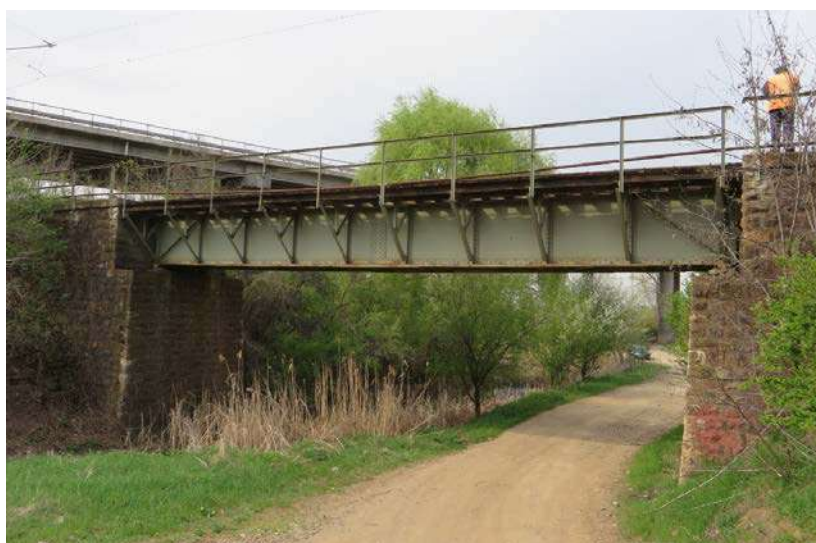
Fig.1. Bridge on the railway line Sofia - Karlovo at km. 22 + 730 near to Jana station
