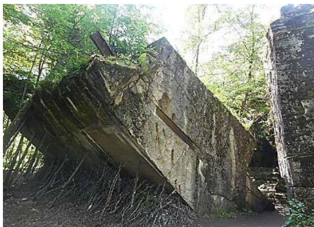
Fig. 15 Separated concrete block of the Göring's bunker (own photo)
