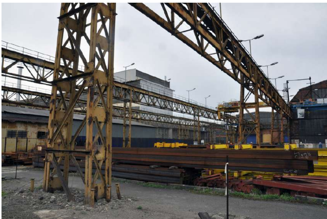
Fig. 1. Steel truss structure supporting an overhead crane
