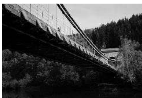
Fig. 9.1 Stadlec Bridge across the Luznice River
