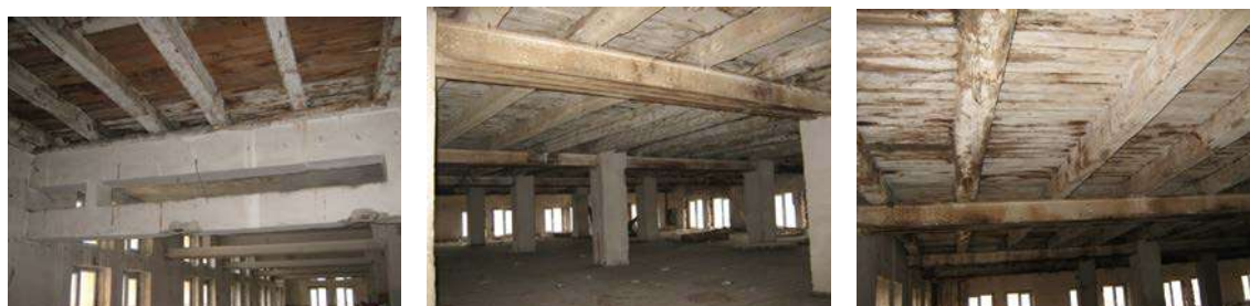
Fig.2.2a,b,c. Supporting of the wooden beams on steel double T- beams; Supporting of the steel beams on the columns of the building.
