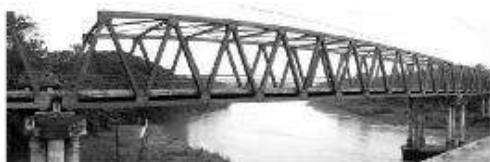
Fig. 22.3 Bantar II Bridge (226 m), Yogyakarta
