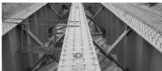
Fig 19.1 Construction of a steel girder bridge Fig. 19.2 I-profile shear studs over the top steel flange.
