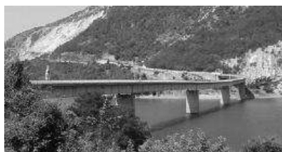
Fig. 14.1 Melnicki Bridge near Debar.
