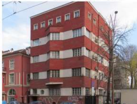
Sofia, 38 "Vasil Levski" Blvd. Building cooperative, 1828-1829.
