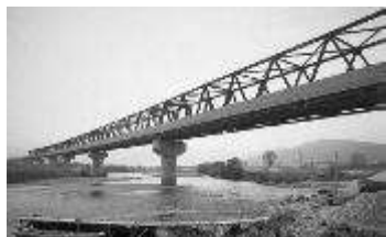
Fig. 24.8 Third Chikumagawa Bridge (Nagano).
