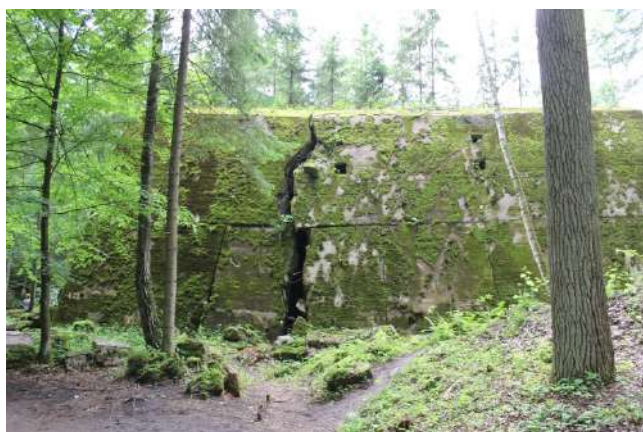
Fig. 14 View of separated but entirely preserved wall of heavy bunkers (own photo)
