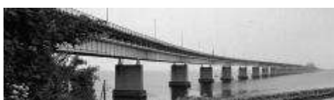
Fig. 10.3 The Storstrøm Bridge from 1937
