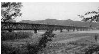
Fig.21. Qiantang River Bridge
