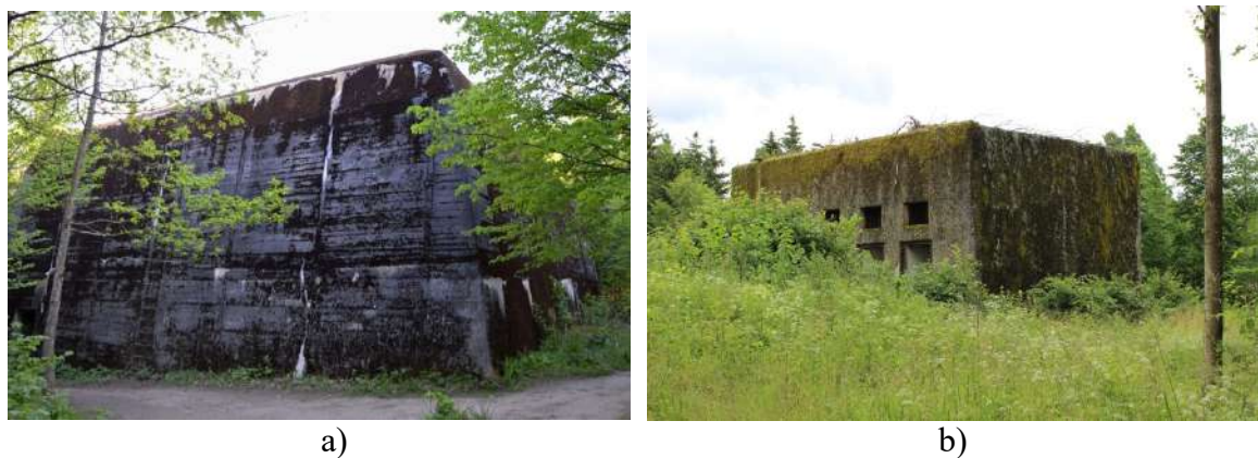
Fig. 13 The entirely preserved heavy bunkers (a) and building of electric transformers (b) in Mamerki.
