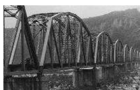
Fig. 25.3 Dajia Creek Bridge
