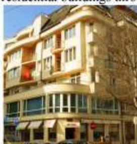
Sofia, 90s. Building with two attic floors
