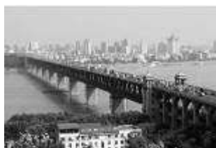
Fig.21.2 Wuhan Yangtze River Bridge
