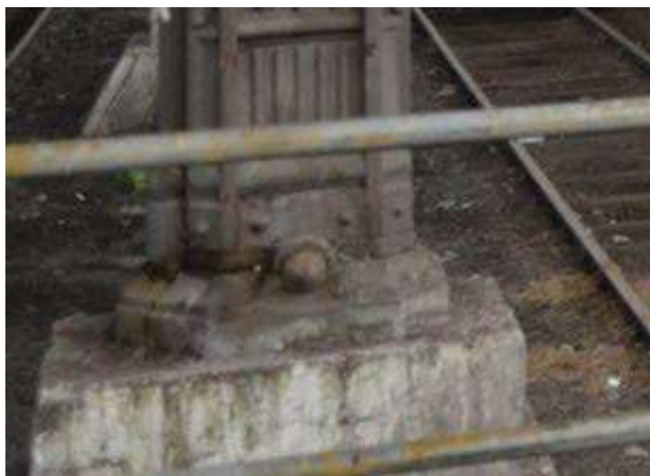
Fig. 6. Hinge at the base of heavy columns (© GOB-DML)
