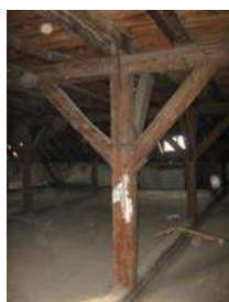
Fig. 3.2a,b,c. Binder, columns (kings) anchored on a binder beam; capitals in the longitudinal direction, slopes to each column; Pliers and kings at each level of the three-storey structure of the roof
