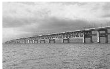
Fig. 24.9 Sky Gate Bridge R (Osaka)
