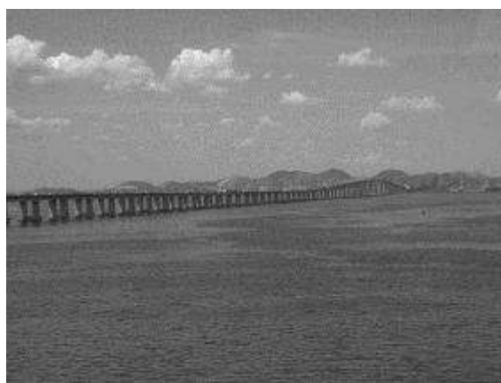
Fig. 5.1 Side view of the Rio-Niterói Bridge.
