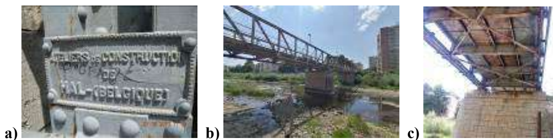
Fig.7.3a,b,c View of a road pedestrian steel bridge on Osam stream
