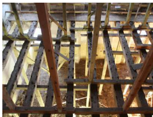
Fig. 3 View of polychrome ceilings, situation 2017, source: Meyer
