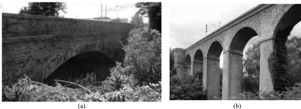
Fig. 3. Analysed bridges (a) single span (b) multi-span [19].
