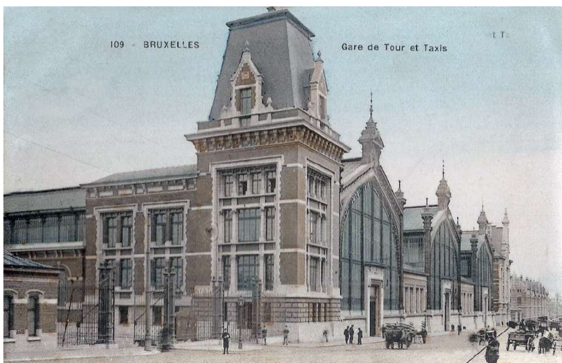
Fig. 9. Outside view immediately after its construction (1910)
