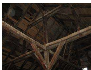
Fig. 3.2a,b,c. Binder, columns (kings) anchored on a binder beam; capitals in the longitudinal direction, slopes to each column; Pliers and kings at each level of the three-storey structure of the roof
