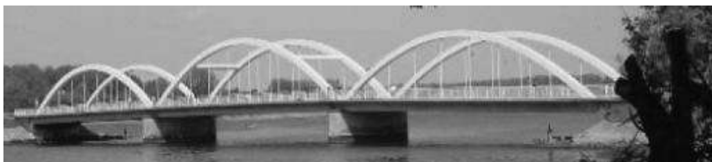
Fig. 10.5 The Munkholm Bridge from 1952.
