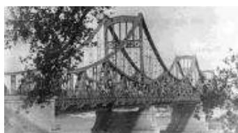
20.6 The rebuilt Mykolaivskyj bridge on old piers
