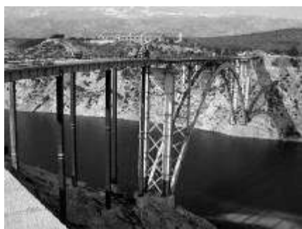
Fig. 8.1 Reconstruction of the Maslenica Bridge for the state road
