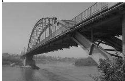
Fig. 23.1 Sefid Bridge in Ahwaz
