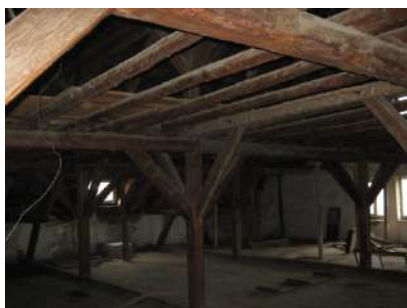
Fig. 3.7. Floor joists of the first new of the spatial structure
