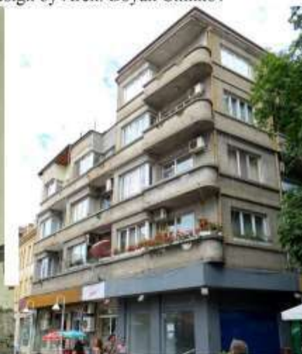
Gabrovo, "General Radetski" Str. Building cooperative, 1930s
