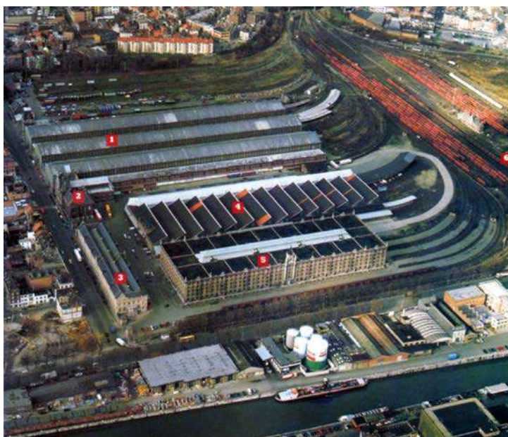
Fig. 1. View from above of former Thurn and Taxis freight station
