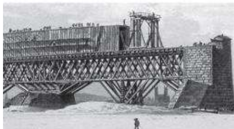
Fig. 2.1.1 Victoria Bridge, Montreal
