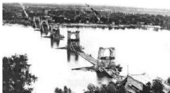
Fig. 20.5 Mykolaivskyj bridge failure
