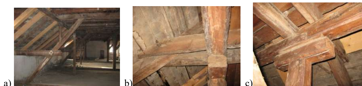
Fig. 3.3a, b, c. Masonry wall attics and inclined beams at the beginning and end of the main spine of the structure
