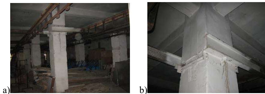
Fig.2.1a,b. Distribution of the columns in the basement of the building-a), View on the floor and column in the first level of building-b)
