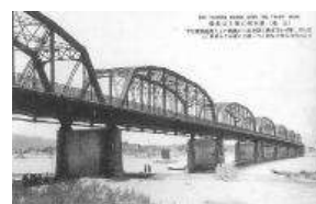
Fig.25.4 Second-generation Taipei Bridge
