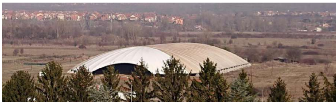
Fig. 3 The second construction phase of the protective structure (2019)
