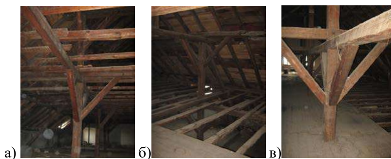
Fig. 3.10a, b, c. View on the second level of the roof structure
