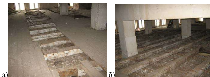
Fig.2.3a,b. View on the beams in the floor construction
