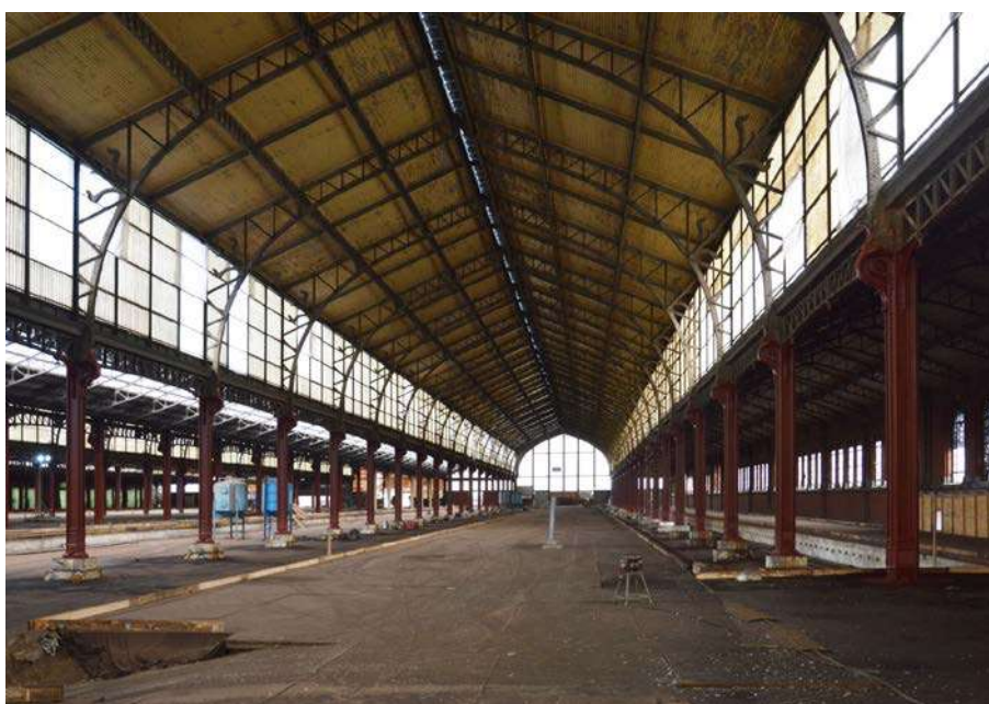
Fig. 4. Inside view of large hall frames (© GOB-DML)
