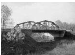
Fig. 15.6a,b,c The first welded steel road bridge in the world erected over the Słudwia River near Łowicz (1929).
