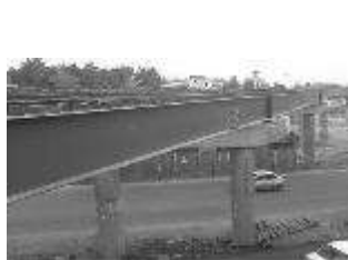
Fig. 23.3 Plate girder bridge
