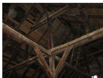
Fig. 3.2a,b,c. Binder, columns (kings) anchored on a binder beam; capitals in the longitudinal direction, slopes to each column; Pliers and kings at each level of the three-storey structure of the roof
