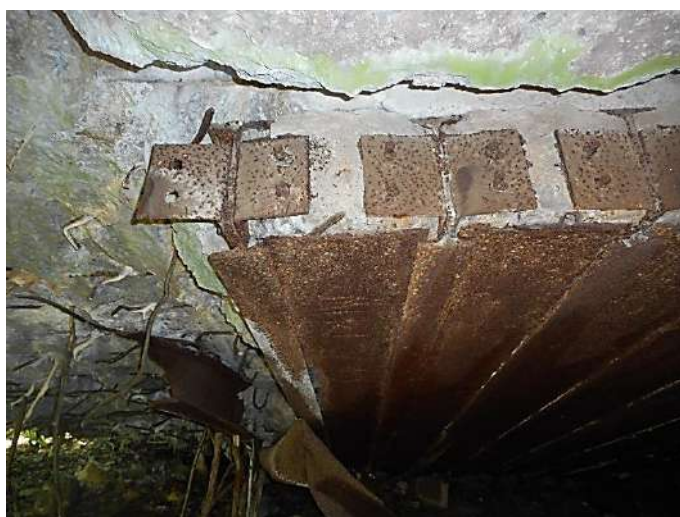
Fig. 7 Composite slab on steel beams (own photo)
