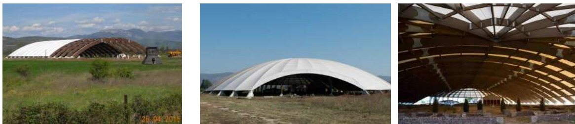
Fig. 4. New Mediana shelter: a) covering progress ; b) look; c) Inside look
