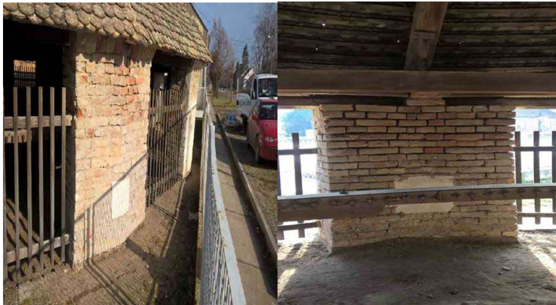
Fig. 8a. Photos remediation short walls
