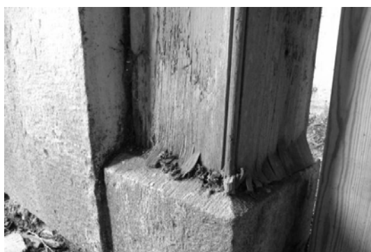
Fig. 20. Brooming at the base of a column.
