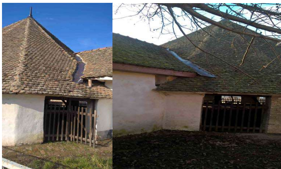
Fig. 7. Rehabilitation of the roof
