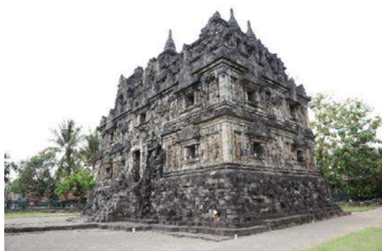
Fig. 7 Heritage building for restoration [3]
