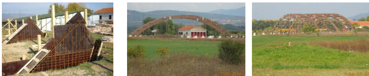
Fig. 3. New Mediana shelter in construction
