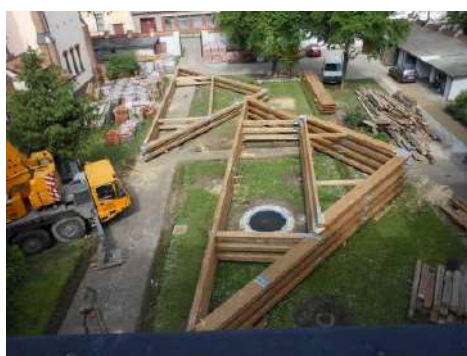
Fig. 20. Main roof trusses construction
