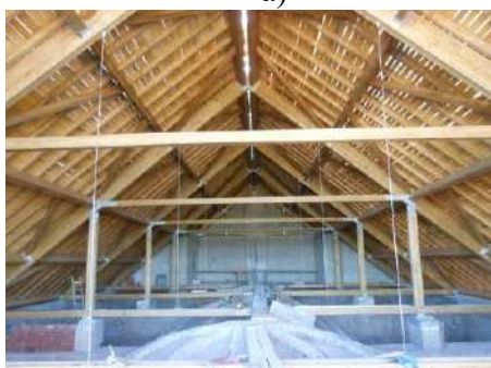
Fig. 21. Part of the completed roof structure from the inside
