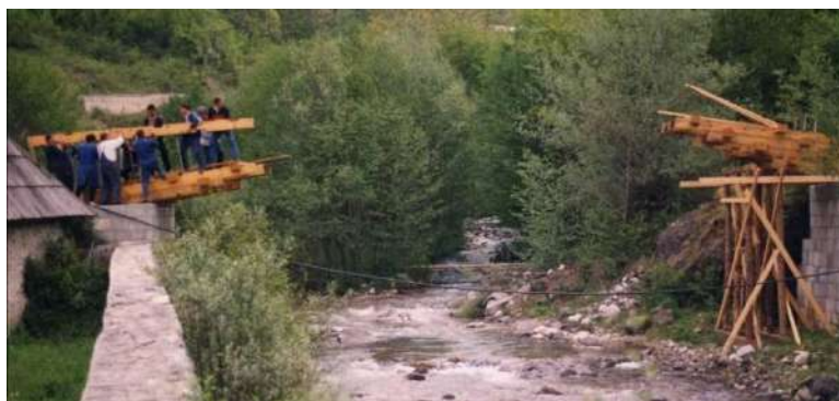
Fig. 8. Bridge in erection stage
