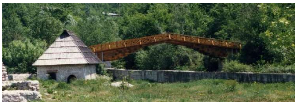
Fig. 9. Completed bridge from the downstream side
