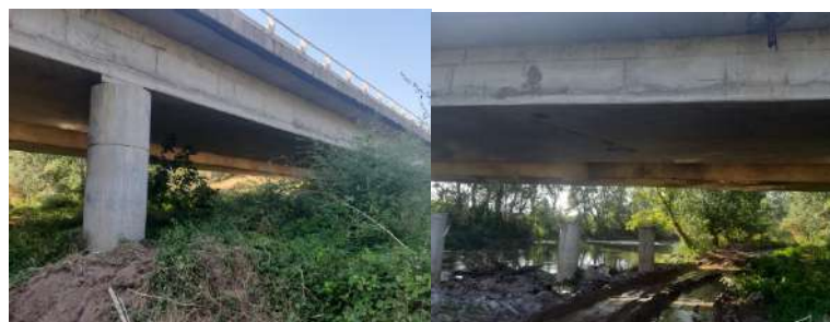
Fig. 21. “L” The highway bridge (incomplete but operating)
