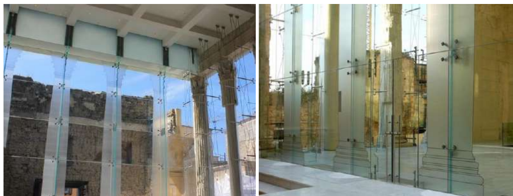
Fig. 18. Float glass restoration of the ruins of the Augustan Temple, Pozzuoli
