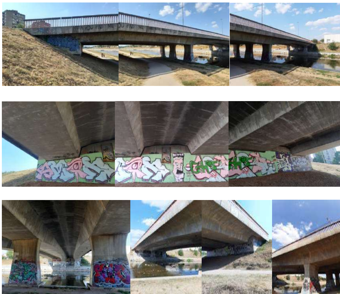
Fig. 11. “H” Chez-Tonic-gas-station bridge
