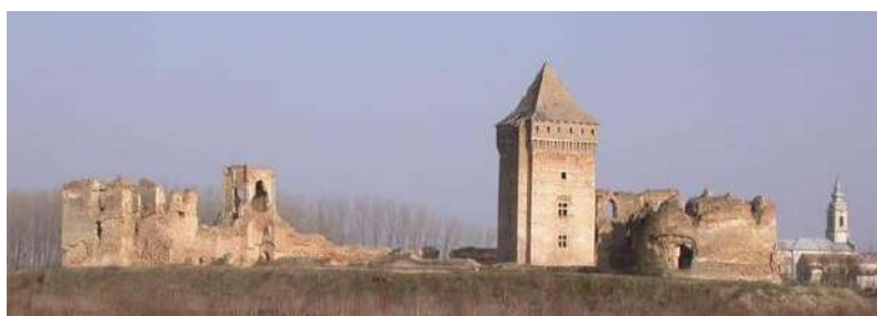
Fig. 2. Bač fortress before the watchtower roof reconstruction
