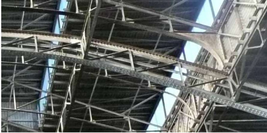
Fig. 10. Connection of top truss to main roof truss
