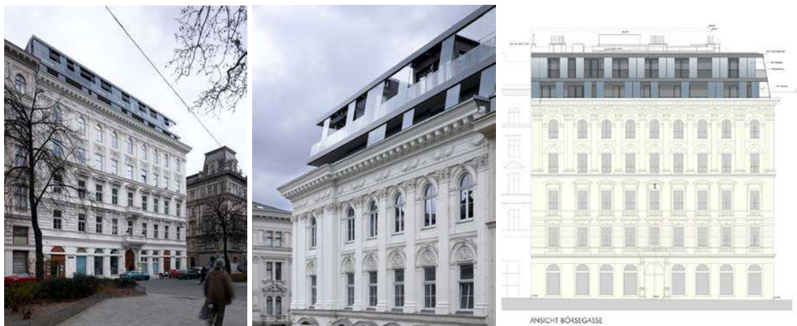
Fig. 2. Roof extension on the stock exchange. Börsegasse 10, Wien, Austria
