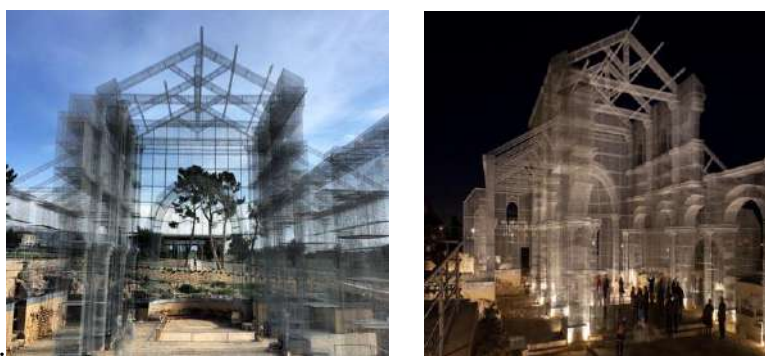
Fig. 14. Restoration with the wire mesh – Basilica of S. Maria Maggiore, Manfredonia ( http://www.italianways.com/a-wire-mesh-paleochristian-basilica/ )
