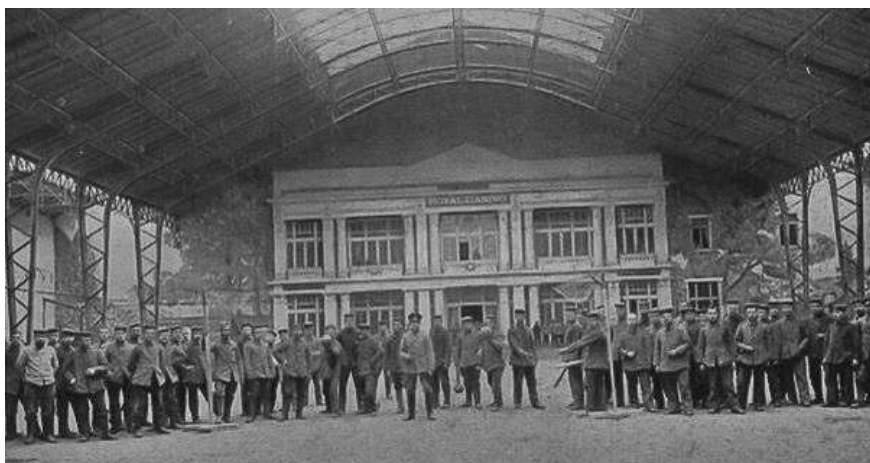
Fig. 10. Photographs taken during construction (top) and early use
