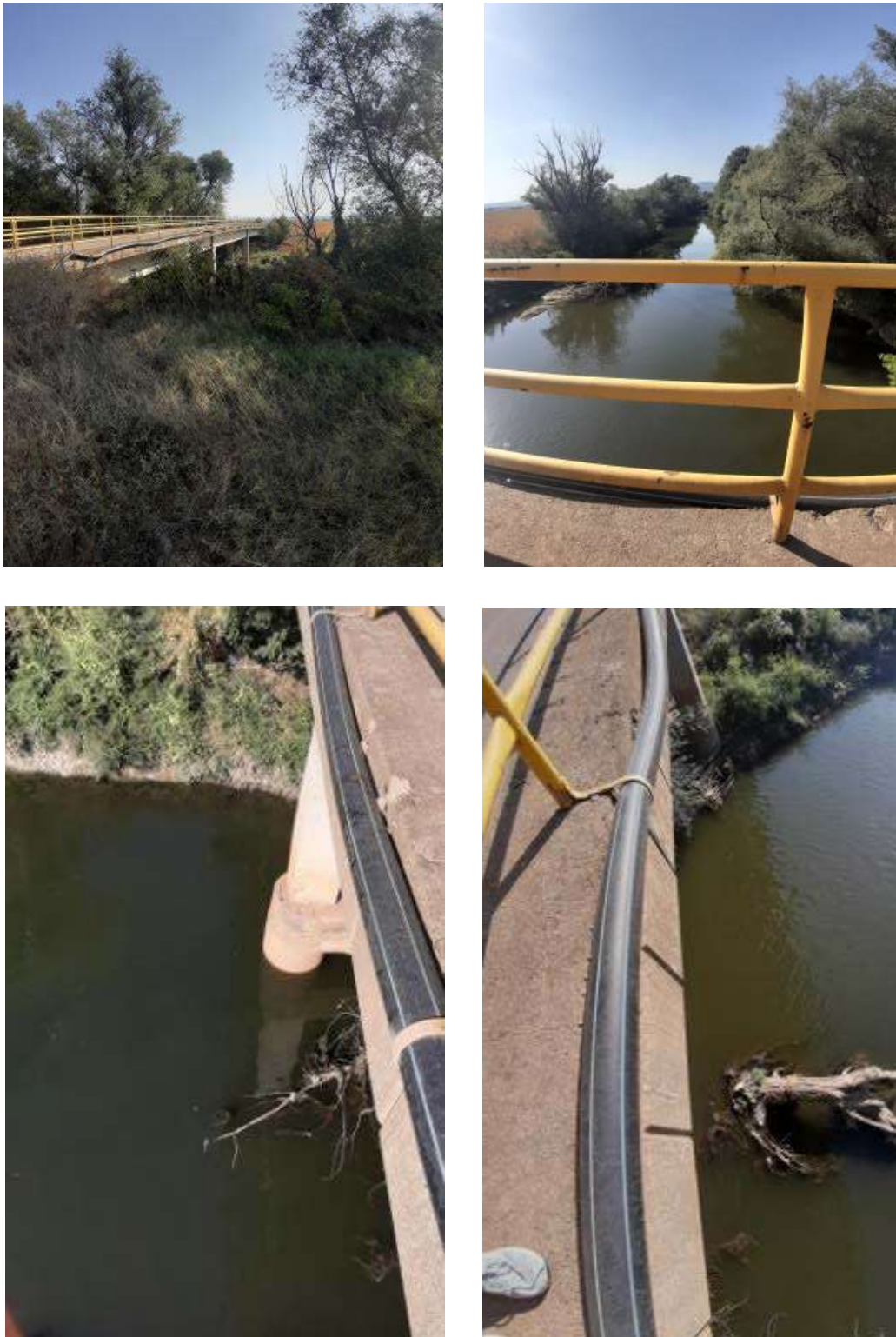
Fig. 22. “M” The last bridge on Nišava in Trupale, Niš
