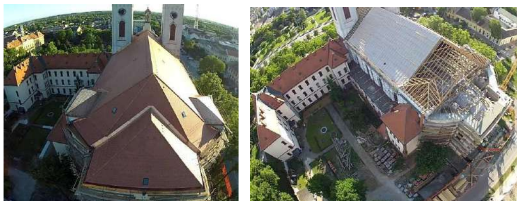
Fig. 23. View of finishing works and completed roof
