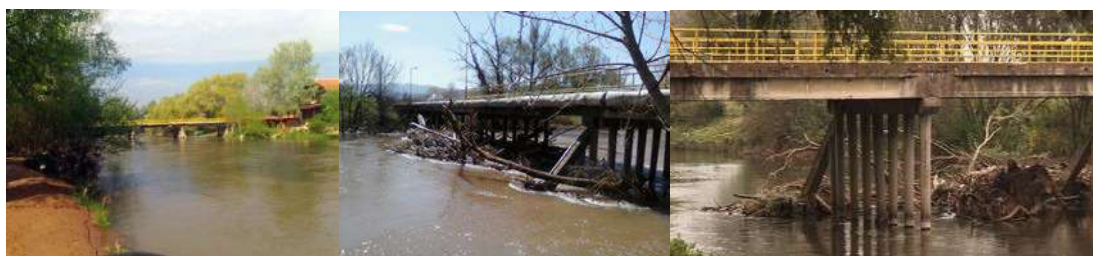
Fig. 7. “D” The Donjovrežinski bridge (in the process of refurbishment/replacement)
