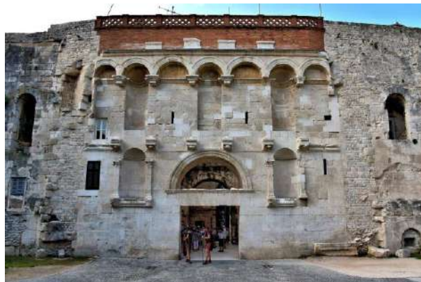
Fig. 10.. Golden Gate of Diocletian Palace, Split – missing part is restored with brickwork
