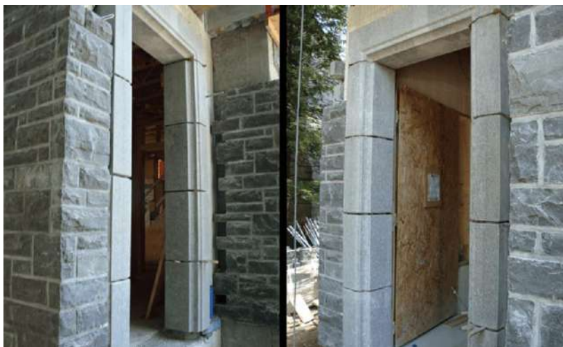
Figure 9. Heritage restoration by using concrete elements ( https://timberhawkhomebuilders.tumblr.com )
