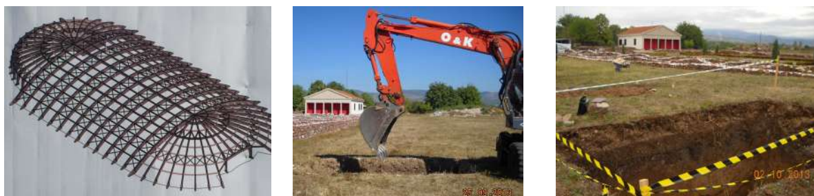
Fig. 2. New Mediana shelter: a) look; b) and c) Excavations for foundations
