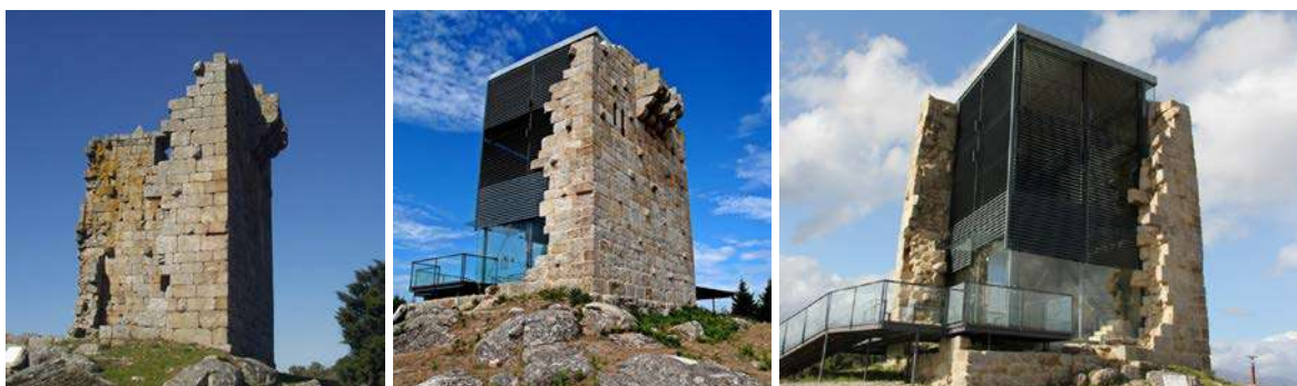
Fig. 10. Tower of Vilharigues before and after restoration, Vouzela, Portugal by Carlos Quevedo Architects
