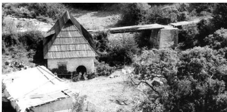
Fig. 7. Provisory structure used for crossing the river before the new bridge construction
