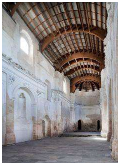
Fig. 11. Wooden barrel vault of the church of S. Maria of Gesù, Modica, Fidone and Messina, 1996. ( https://www.bta.it/txt/a0/06/bta00699.html )
