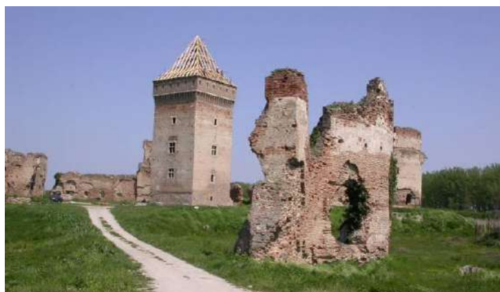
Fig. 5. Final works on roof reconstruction
