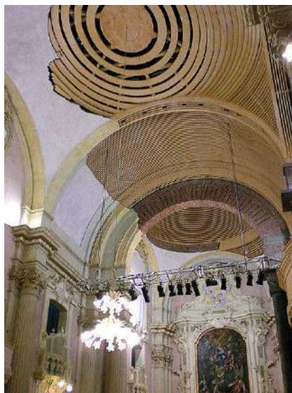
Fig. 11. Wooden barrel vault of the church of S. Maria of Gesù, Modica, Fidone and Messina, 1996. ( https://www.bta.it/txt/a0/06/bta00699.html )
