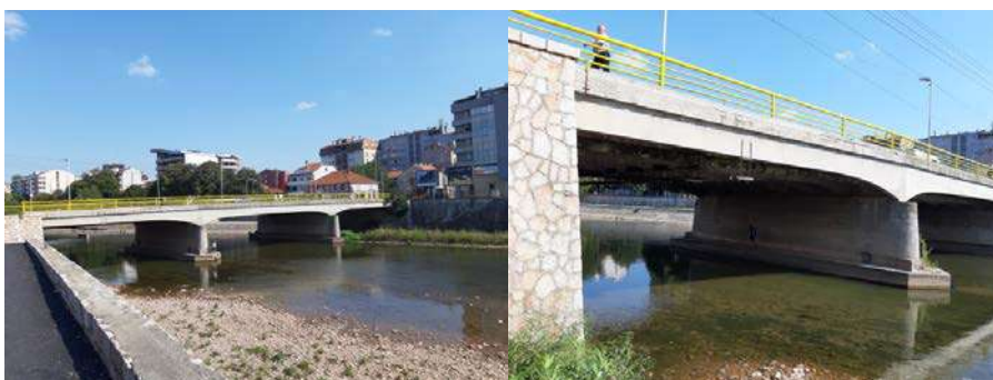
Fig. 15. The Stone Bridge
