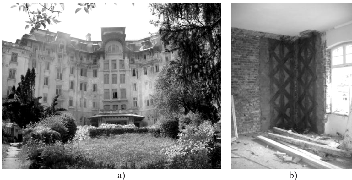
Fig. 5. Combined EBR and Central core strengthening techniques applied to: a) Palace Hotel, Govora; b) FRP EBR and central core reinforcements applied on an URM wall [20]
