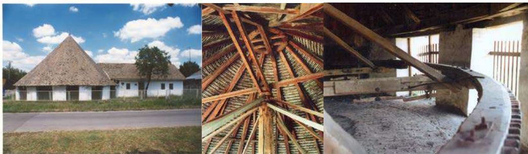
Fig. 1. Photos dry mills appearance, the roof wooden structure with pillar „popa,, i craft wooden structure
