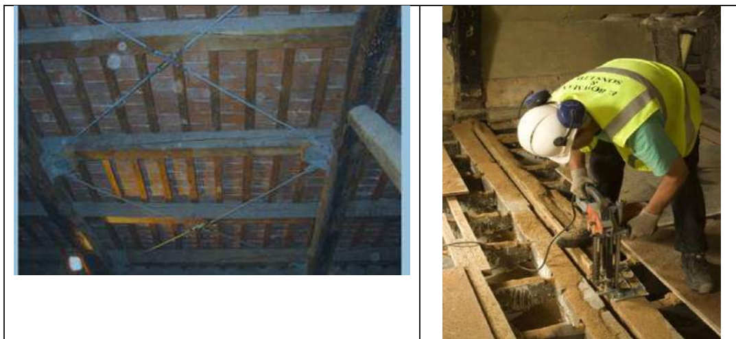
Fig.6. Visible and hidden use of steel elements for reinforcement of the floor beams
