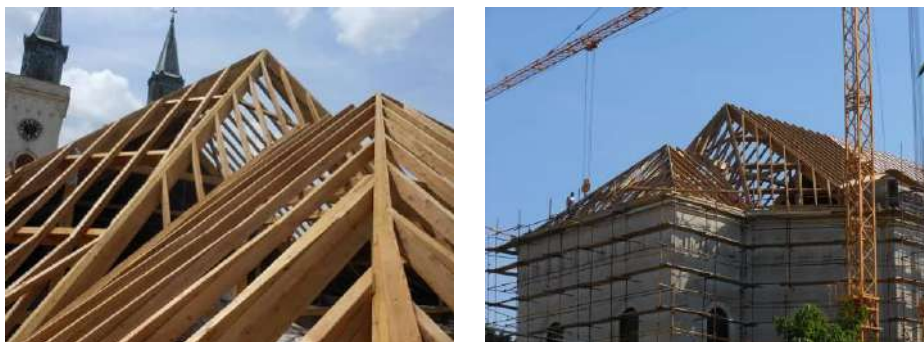
Fig. 22. Works on the roof part above the church alter
