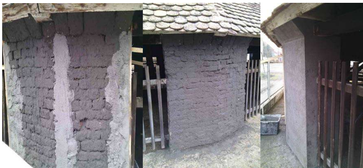
Fig. 8b. Photos remediation short walls
