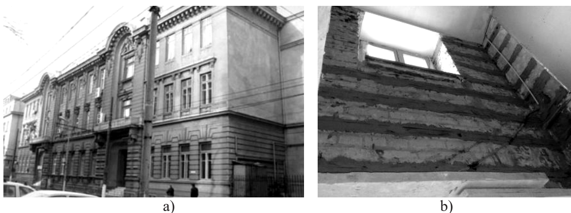
Fig. 2. FRP EBR strengthening technique applied to: a) Victor Slăvescu historical building; b) Laminates bonded on an URM wall [20]
