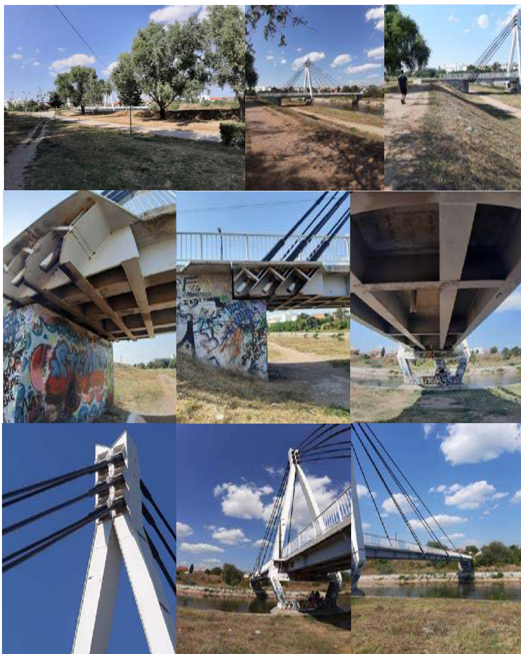
Fig. 10. “G” Pedestrian Bridge
