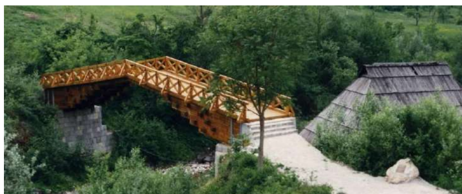
Fig. 10. Completed bridge from the upstream side
