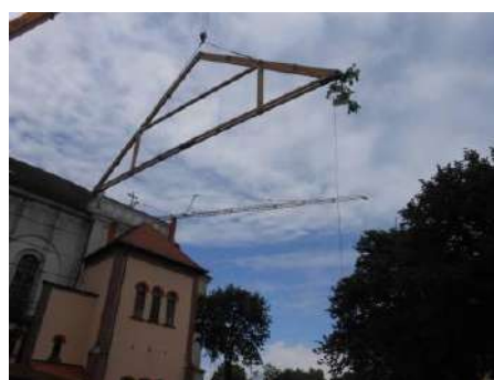
Fig. 20. Main roof trusses construction
