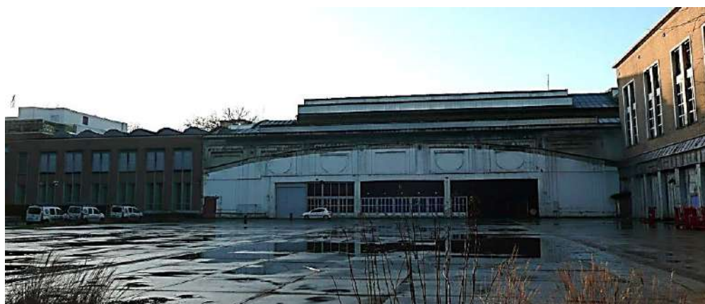
Fig. 1. Cemented North façade of the Floralia Hall
