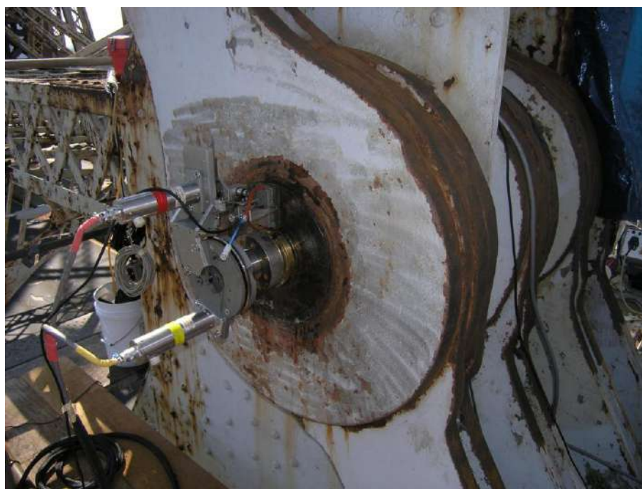
Fig. 5. Phased-array ultrasonic testing of a pin
