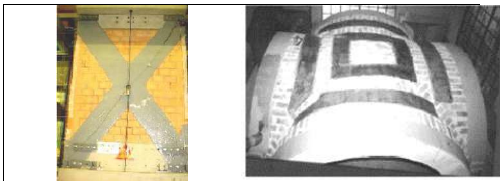
Fig. 8. Different uses of FRP reinforcement (after [1])
