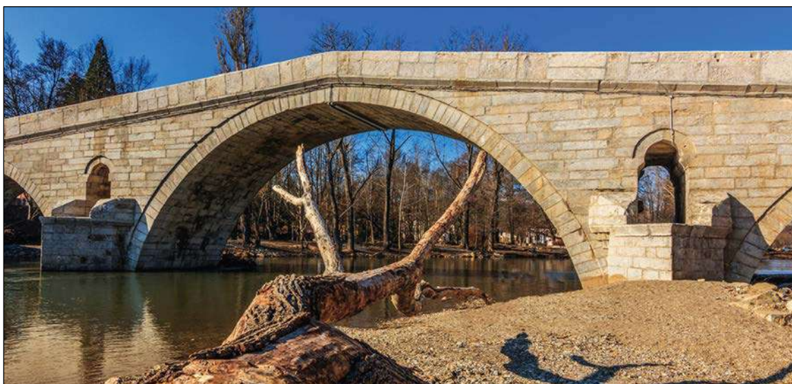
Fragmentary view from the central part of the hull of Kady Bridge with the specific vaultings and clogging protection of the relief openings
