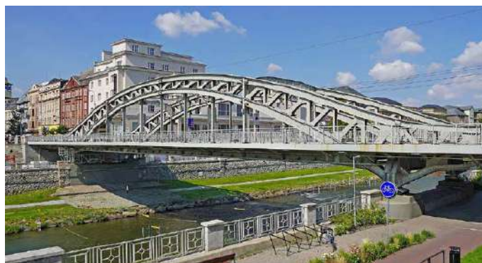
Fig. 36. A road bridge over the River Ostravice with a three-span bridge of the Gerber beam-type with span lengths of 16+60+16 m, from 1914[20]
