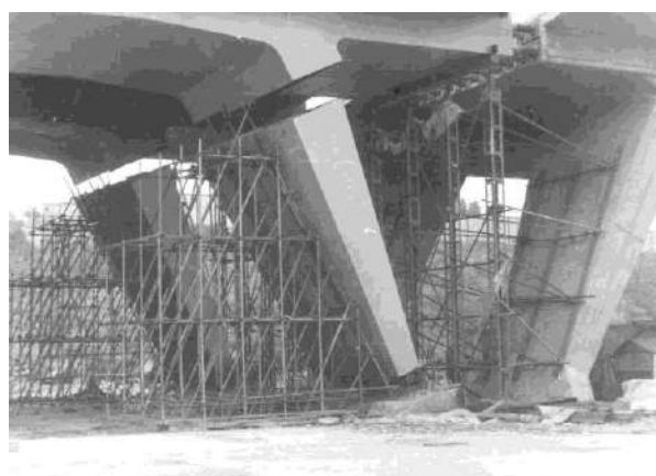
Fig. 7. Assembling of the steel “V”-supports
