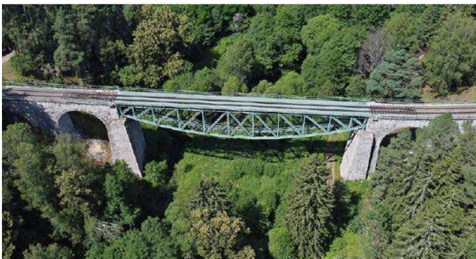
Fig. 34. The railway bridge near the village of Čistá; in the mid-span there is a steel beam truss bridge with a lower parabolic chord, span 57.0 m, from 1898 [20]
