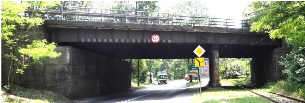
Fig. 1 The considered viaduct seen from the side of Tarnopolska Street.
