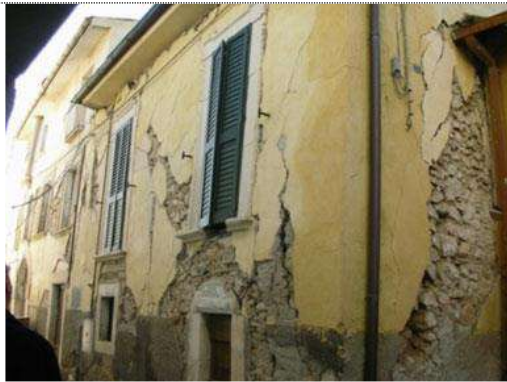
Fig. 11. Severe damages to shear walls and spandrels 2009 Eq. L'Aquila, Italy, [22]
