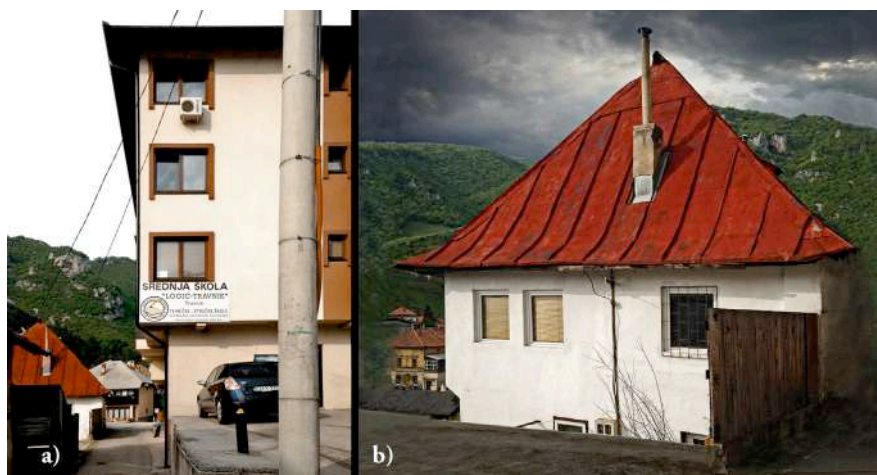
Fig. 4. An inappropriate modern intervention in a historical setting. a) High school in Osoja where one of the traditional residential houses in the Osoja settlement is visible on the left. b) Traditional residential house in the settlement of Osoja. Status recorded in May 2014.
