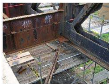
Fig. 19. Truss joint with double-walled lower chord[20]
