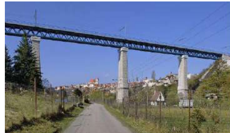
Fig. 26. Truss half-through bridge with upper parabolic chord (road bridge to Císařská louka from 1901)[20]
