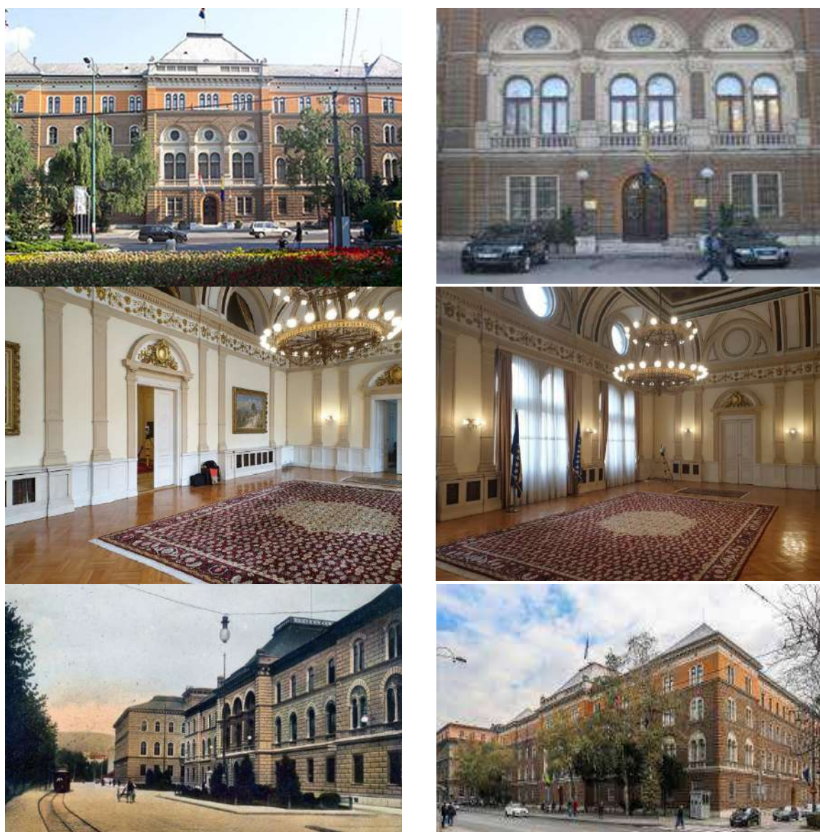
Fig. 3 Royal Administration building of Drinska Banovina in Sarajevo
