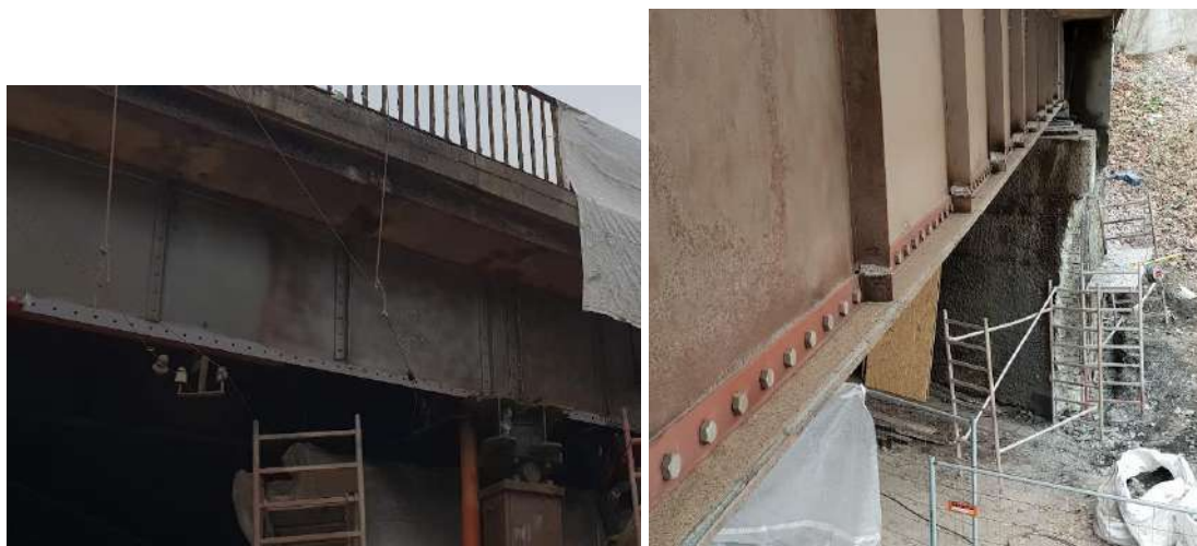
Fig. 17. The girder number 8, including: on the left - condition after removing the angles and the sheets forming the bottom flange, on the right - condition after inserting the new angles and the new bottom flange.
