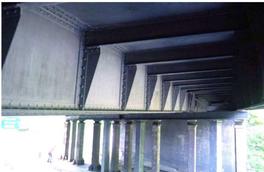
Fig. 6 Construction of the intermediate support of the viaduct (The cross beam crowning the row of steel pillars is noteworthy. The ribbing of the main bridge deck girder is also visible in the foreground).
