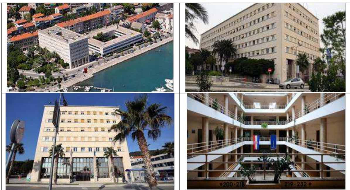
Fig. 9. Royal administration building of Primorska banovina
