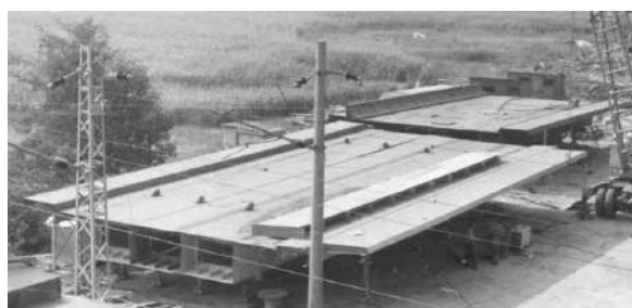
Fig.3. Triple-box section of the bridge deck
