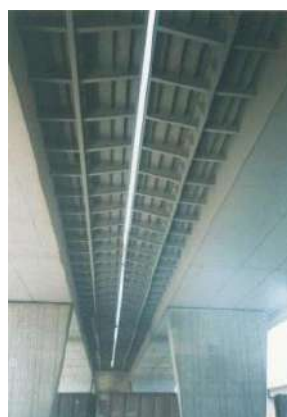
Fig. 9. A view from beneath the steel orthotropic bridge
