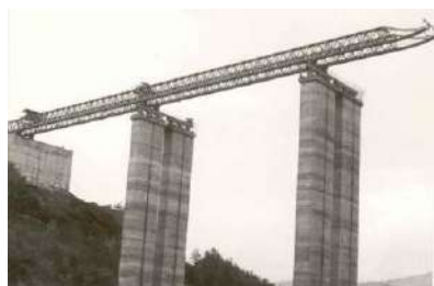
Fig.10e,f. Overall view of the steel trusses – e); Cross-Section 3-3 and 4-4 of the two Trusses – f)
