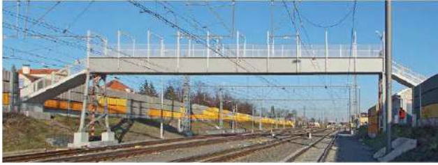
Fig. 22. Plate girder bridge with half-through bridge deck (footbridge in Prague Hostivař from 1937)[20]
