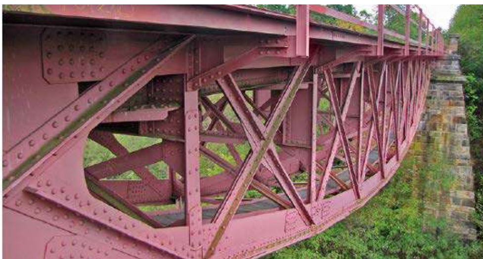
Fig. 32. Railway bridge over the Klabava valley. Steel semi-through truss bridge with parabolic lower chord from 1892[20]
