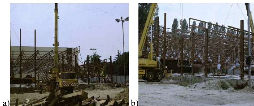
Fig.15a,b. Assembly - view: north –a); Installation - view: west –b)
