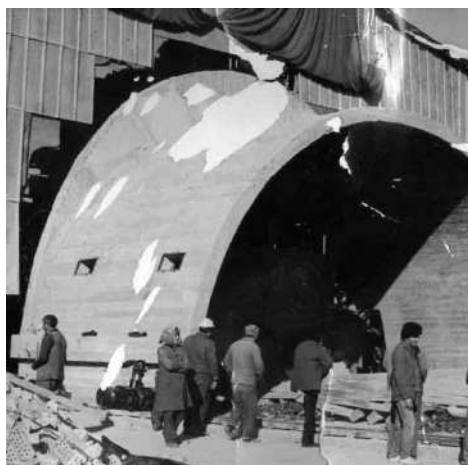
Fig. 21. Covering shell structure at the site
