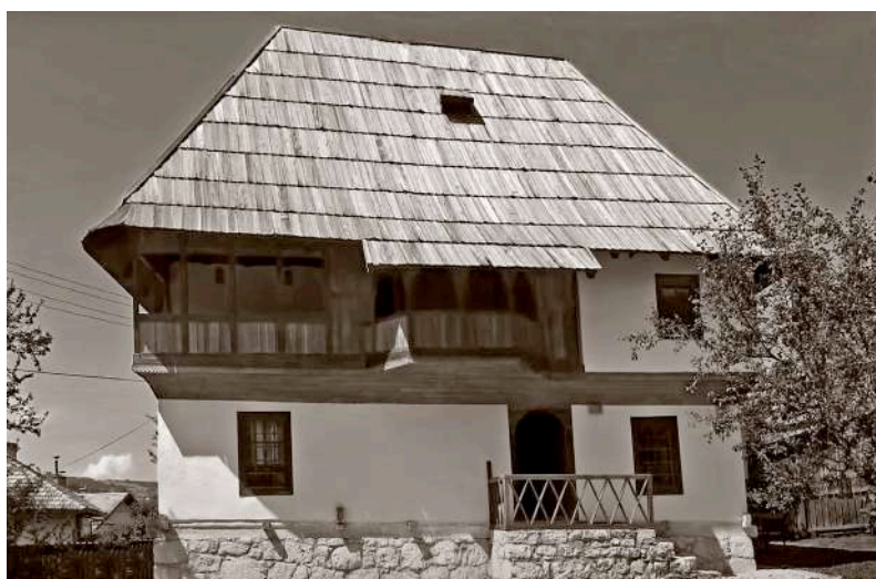
Fig. 14. Čardaklija , built before 1840. years, surroundings of Travnik.
