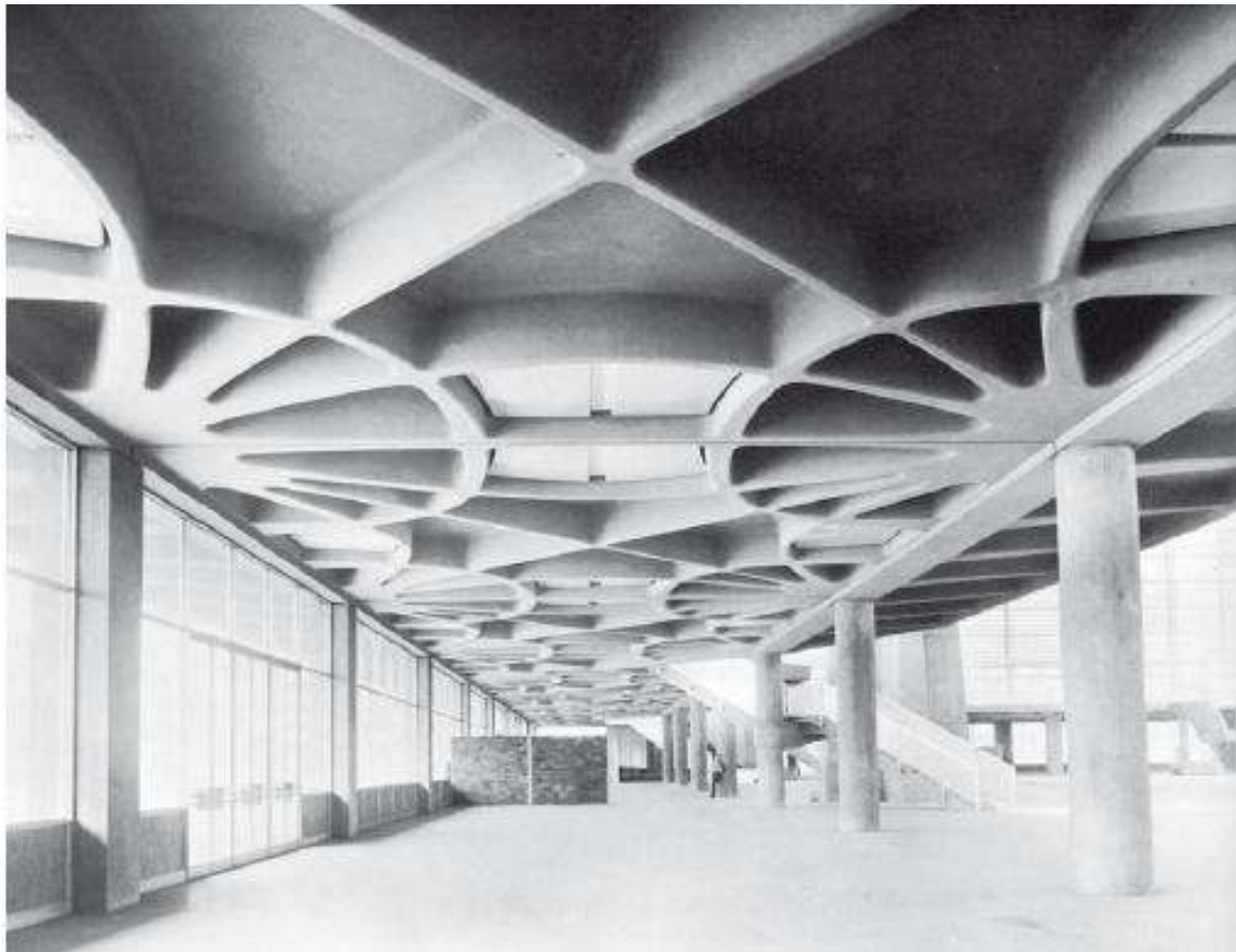
Fig.20. The original ceiling with isostatic ribbed slabs
