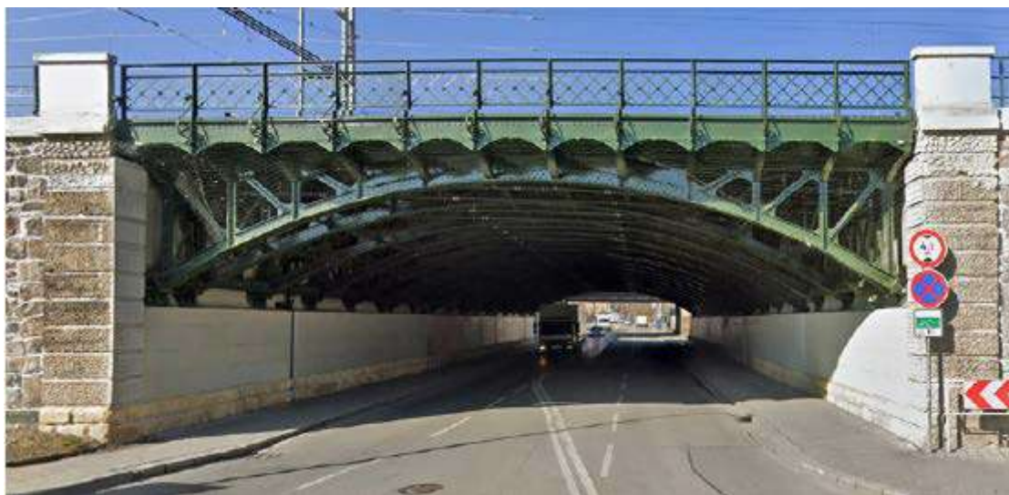
Fig. 33. The railway bridge over Hybešova Street with one span of 15.2 m, from 1897[20]
