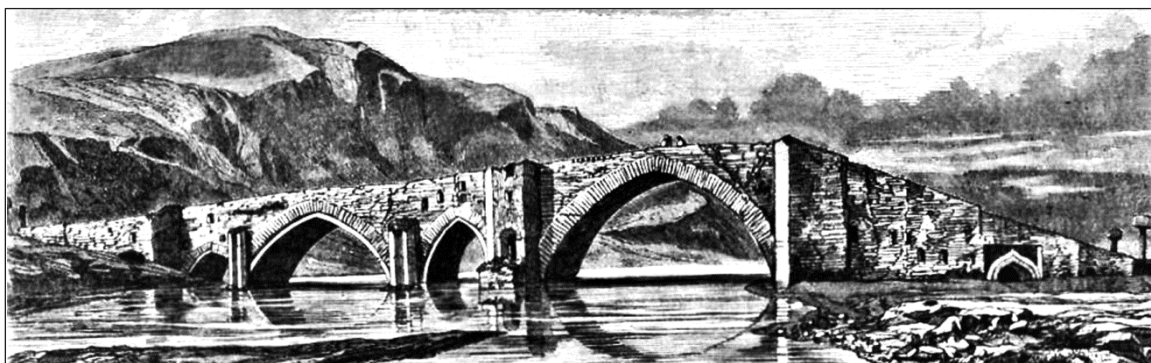
The Azerbaijani Red bridge (Qırmızı Köprü, Sınıq köprü – The broken bridge, 12th century, reconstructed in 1647) over the Efram river (Georgian – Hrami) near Julfa, Lower Kartli (Azerbaijani – Nahicevan)
