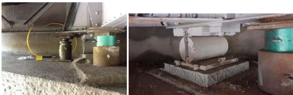
Fig. 15. The repair details of the support bearing, including: on the left - temporary lifting of the bridge deck by means of the hydraulic actuators, on the right - shifted bottom plate of the bearing with a new bearing pad.
