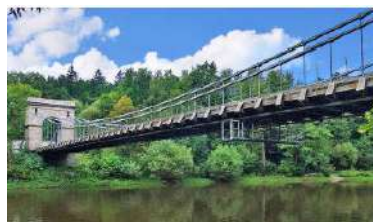
Fig. 2. Suspension bridge in Stádlec[20]
