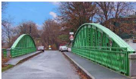
Fig. 26. Truss half-through bridge with upper parabolic chord (road bridge to Císařská louka from 1901)[20]
