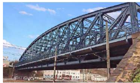
Fig. 24. Truss half-through bridge with straight chords (railway bridge in Prague under Vyšehrad from 1871)[20]
