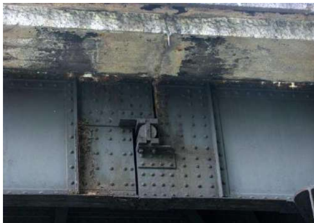
Fig. 5 Riveted construction of a hinge within the main girder.
