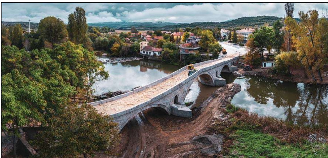
Photogrammetric façade plan of Kadiyski (Kadin) Bridge – NINCH archive; view from the bridge during restoration activities in 2020
