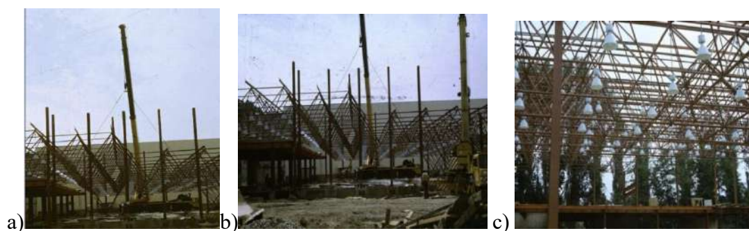
Fig.14a,b,c. Technology of installation of the steel structure
