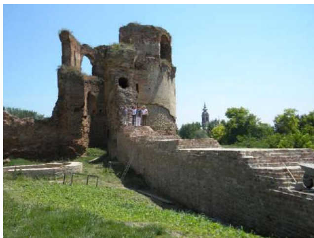
Fig. 3: The tower of Bač as practical example of minimum intervention after works (photo by Nedeljko Markovic)
