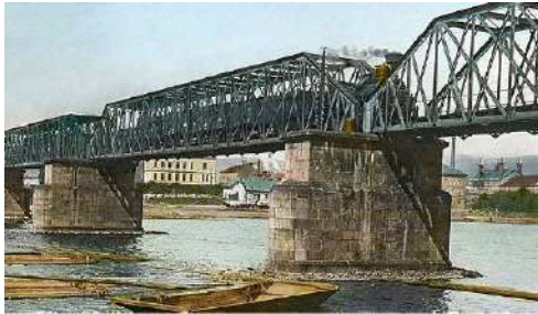
Fig. 24. Truss half-through bridge with straight chords (railway bridge in Prague under Vyšehrad from 1871)[20]
