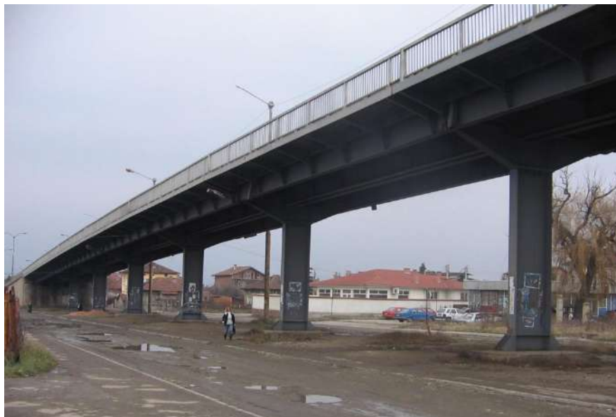
Fig. 23. The completed bridge
