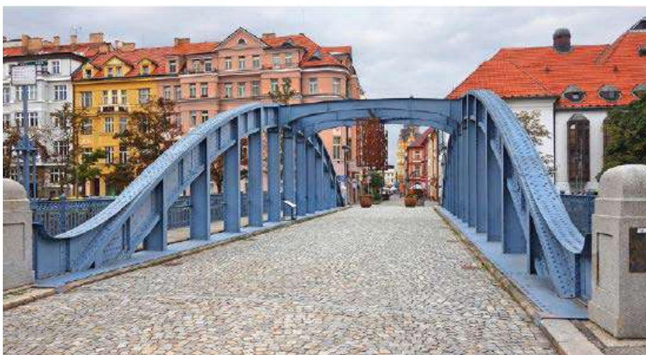
Fig. 35. A road bridge over the River Malše with one span of approximately 40 m., from 1915[20]
