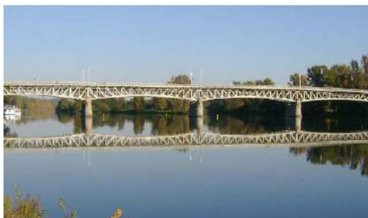
Fig. 28. A truss semi-through bridge with variable height of main girders (Gerber beam). (Tyrš road bridge over the River Labe in Litoměřice dating from 1910)[20]
