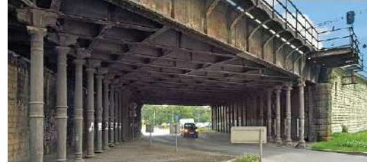
Fig. 22. Plate girder bridge with half-through bridge deck (footbridge in Prague Hostivař from 1937)[20]
