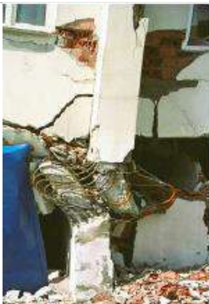
Fig. 3. Collapse with column shear and axial failure. Koceali Eq. 1999.
