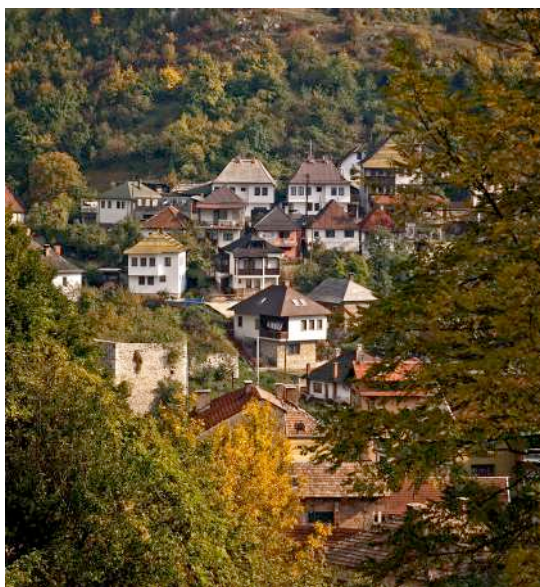
Fig. 17. Typical 'mahala' (city District) - scene Osoja. One-story residential building with a southern facade facing a greater slope.
