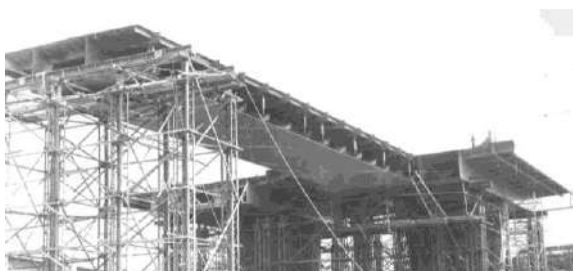
Fig. 4. Assembly of the box girders
