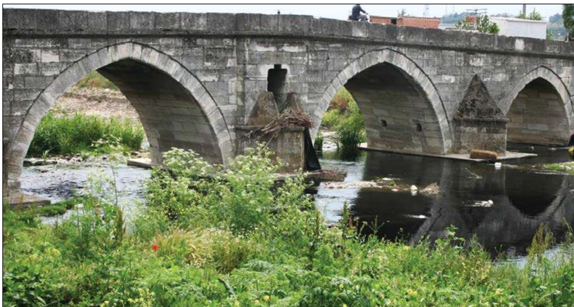
Sokullu Mehmet Paşa Bridge (15th century) in Lüleburgaz, Kırklareli province (Bulgarian name – Lozengrad). Photographic views from the end of 19th century on a marked superstructure plan by Bozkurt (1950), and current condition
