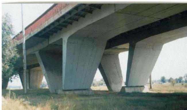
Fig. 8. A view of the concrete and steel bridges
