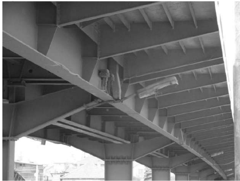
Fig. 22. View of the sidewalks of the completed bridge (bottom).
