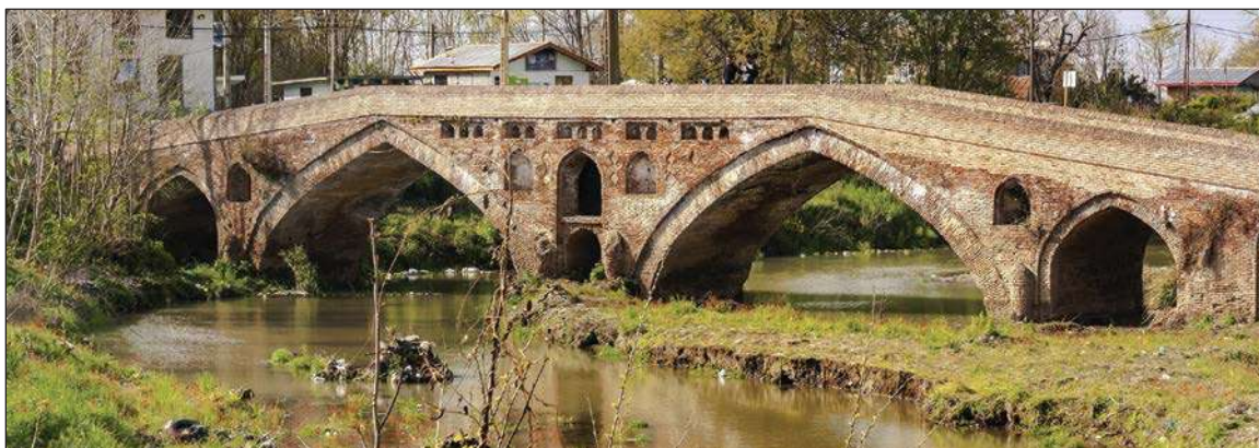
The Iranian brick bridge Pol-e Tamijan (1354/5) over the Tamijan river near Rudsar village, Gilan province, Iran
