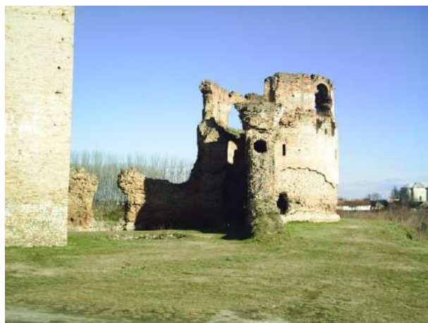
Fig. 2: The tower as practical example of minimum intervention before works (photo by Nedeljko Markovic)
