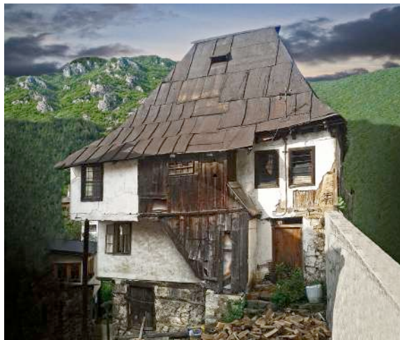
Fig. 18. The building is located in Donje Osoje street, built in the Ottoman period. View of the entrance (western) facade. Condition of the facility in 2014.
