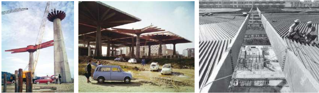
Fig.7. The construction of the “umbrellas”
